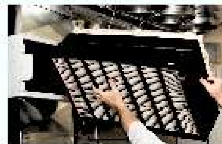
HVAC System comprising with HEPA filters
